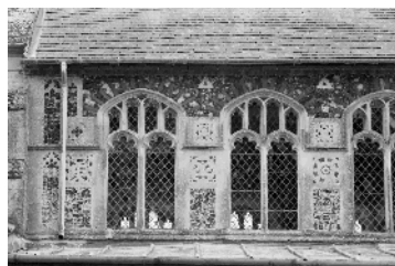
Clerestory windows after repairs
